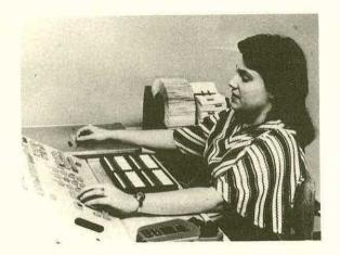
Figure 1. Operator at braille display equipped TSPS console. The abacus and Banks braille writer have been replaced by braille scratchpad.
