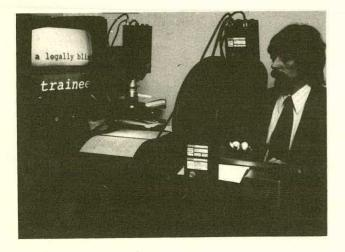
Figure A-3 Employee Typing Document From Copy With Aid of CCTV Selectric System
